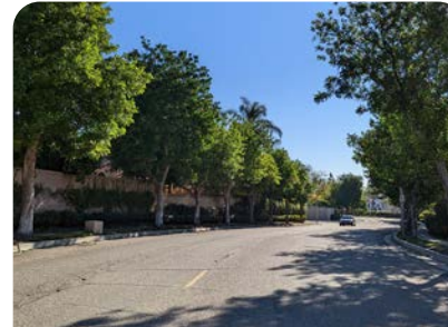
Wide travel lane widths along Mountain View Dr. can provide buffered bike lanes
