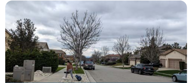
A curb ramp with tactile bumps can improve ADA access for pedestrians traveling across Stoneview Rd. to the neighborhood paseo
