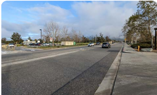
Buffered bike lanes on East Ave. can provide more comfortable bicycling facilities near Summit Intermediate School, Etiwanda Colony Elementary School, and Etiwanda Creek Community Park.
