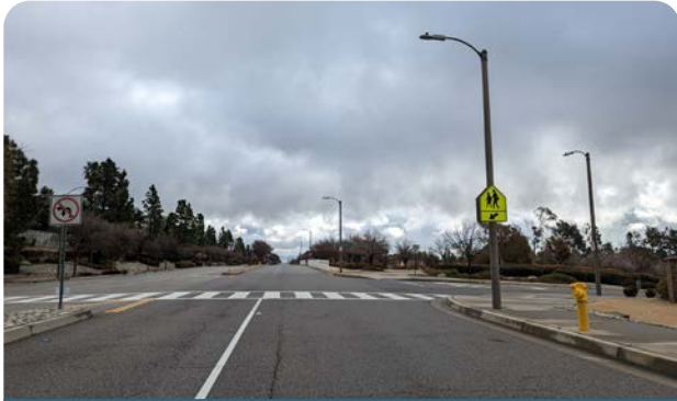
Wide travel lanes on Wilson Ave. can provide buffered bike lanes that increase comfort for bicyclists
