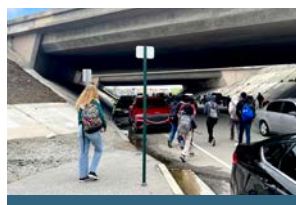
Discontinuous sidewalk traveling under Interstate 15. ↴ Etiwanda High School
