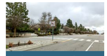
Multi-lane roadway crossing missing pedestrian curb ramps. ↴ John L. Golden Elementary School
