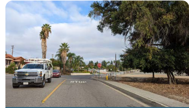
Existing asphalt sidewalks near Valle Vista Elementary
