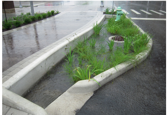
Storm infiltration system in bulbed corner
