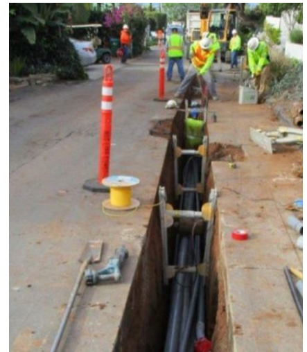
Work to underground utility poles and wires
