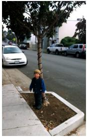
Parking lane planters can be a continuation of the sidewalk curb, or be constructed separate from the curb.
