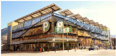
Parking structure artfully screened, and shaded with solar panels
