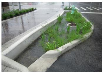
Storm infiltration system in bulbed corner
