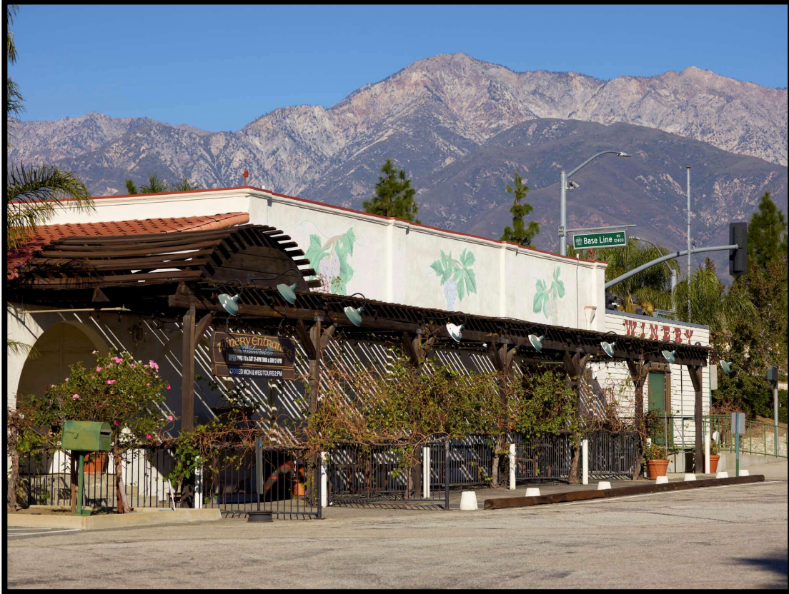
East Elevation of Winery Building
