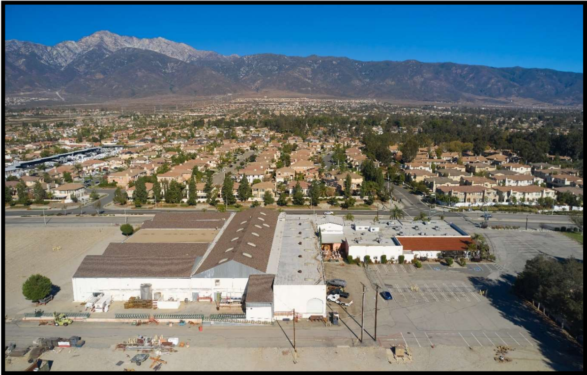
Overhead View of Winery Building Looking North
