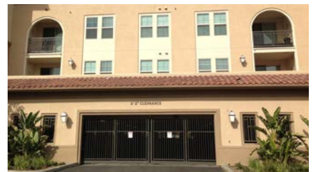
Window openings allow natural light & ventilation
