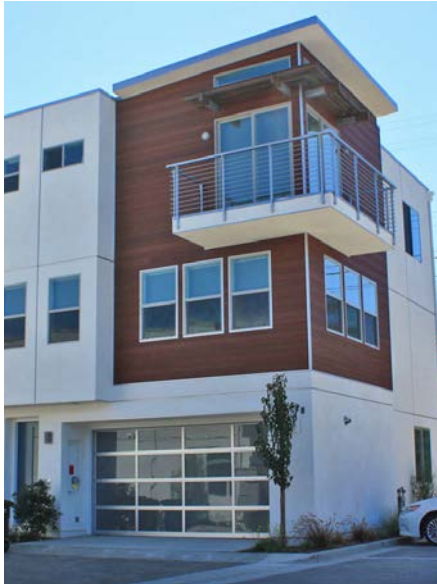
Recessed garage conditions with upper story projections
