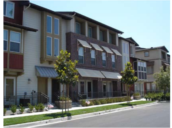
Composition of roof forms, projections, and awnings
