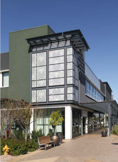
Development standards are designed to maximize creativity and flexibility in design to create active people places.
