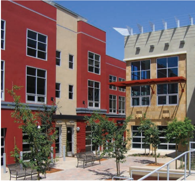
Variation in parapet height, design, and materials with central common open space
