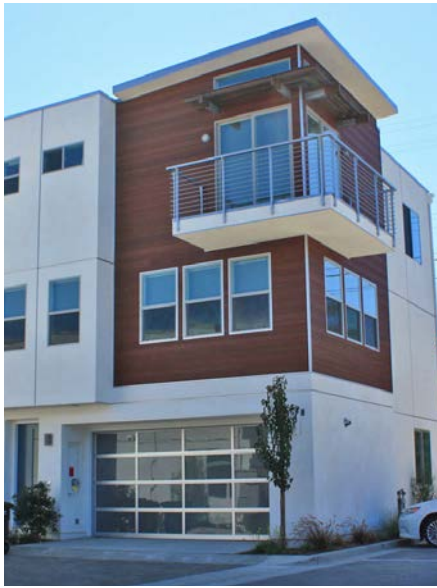
Recessed garage conditions with upper story projections
