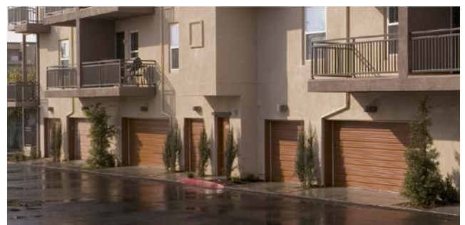
Upgraded garage doors, projecting private open space, and color blocking enhance the private drive aisle experience
