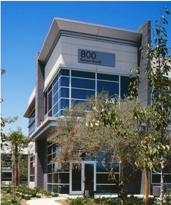
Massing, materials, and glazing activate non-residential corner
