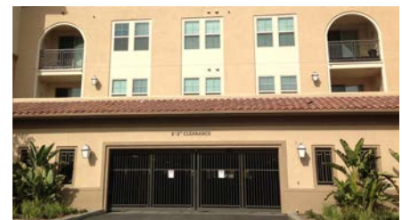
Window openings allow natural light & ventilation
